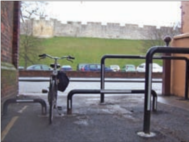
Figure 8.7 Barrier with wheelchair bypass (Tim Pheby)
