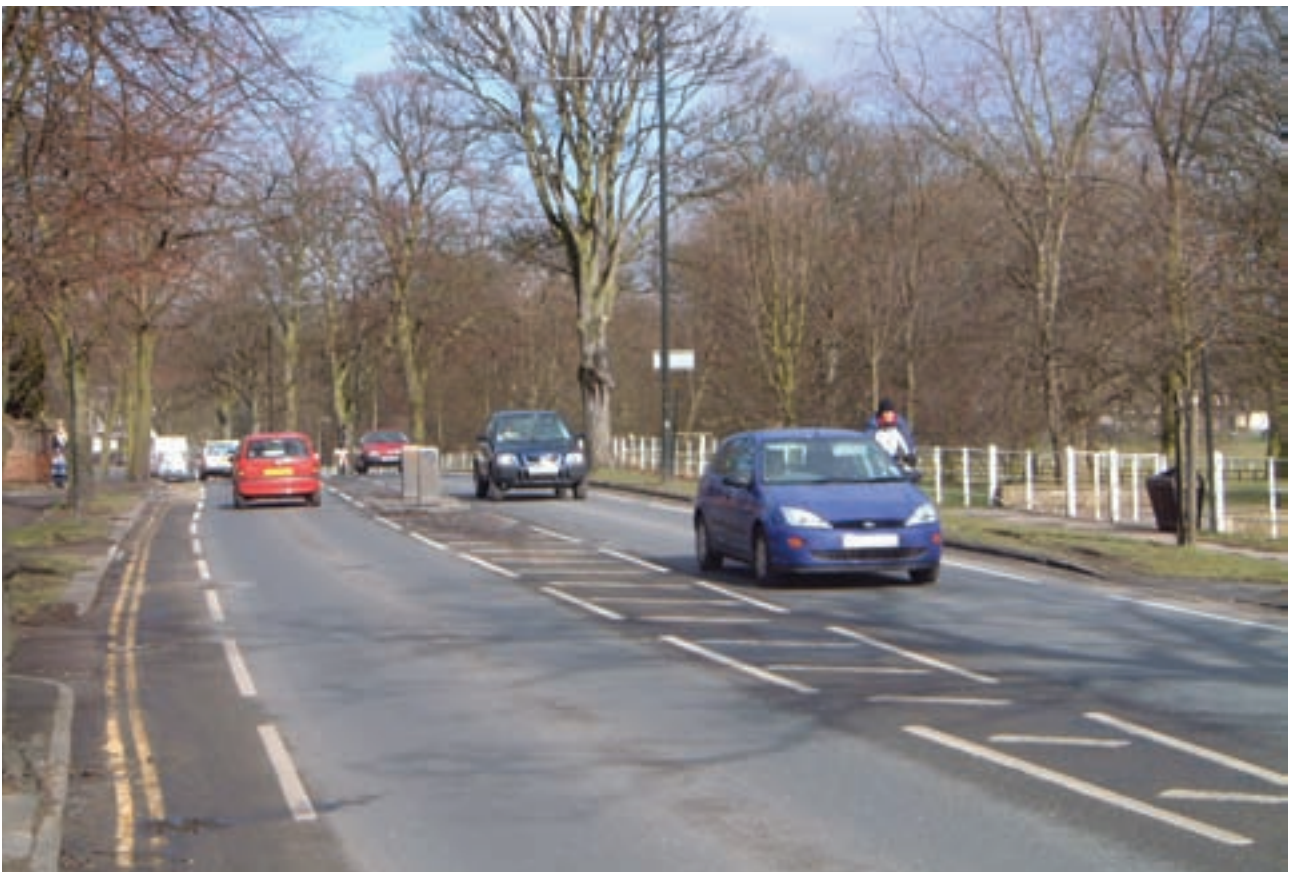
Figure 5.5 Cycle lane continued at refuge (CTC Benchmarking)
