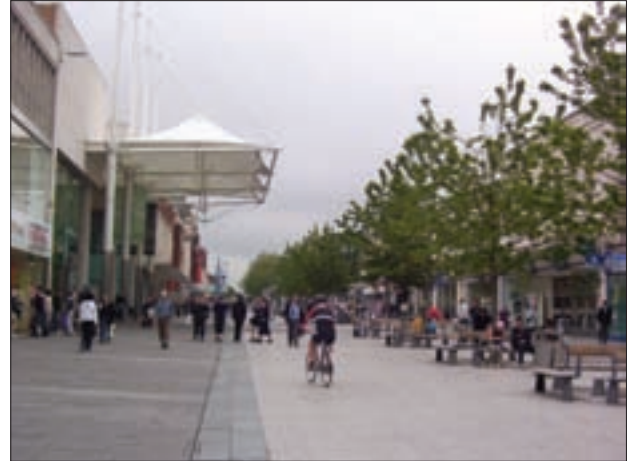
Figure 4.6 Contrasting surface treatments used to suggest where cycling may be more appropriate (Patrick Lingwood)
