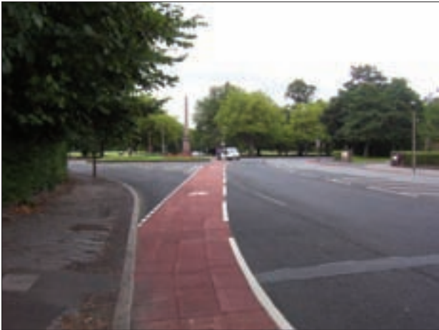
Figure 7.4 Coloured advisory cycle lane crossing side road junction (Steve Essex)
