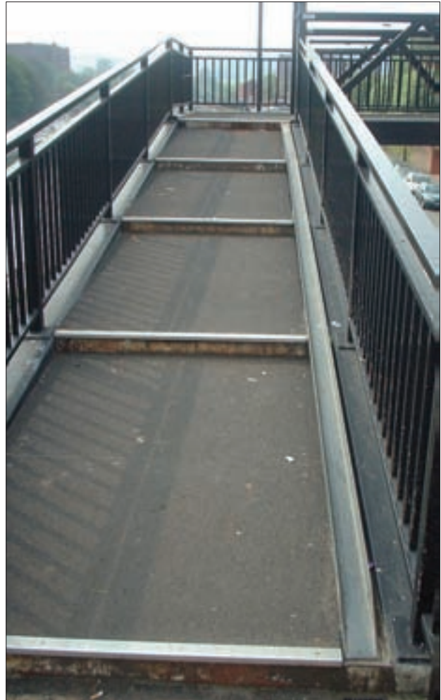
Figure 10.11 Channel section wheeling ramp fitted to existing footbridge (Adrian Lord)
