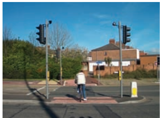
Figure 10.8 Toucan crossing with central refuge and nearside aspects (Alex Sully)
