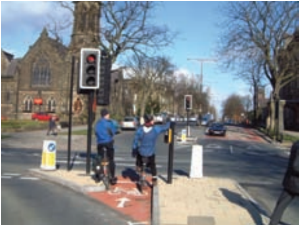
Figure 9.4 Cycle-only phase at signal controlled junction (CTC Benchmarking). Note that the signal head is incorrect, as it uses a red cycle symbol.
