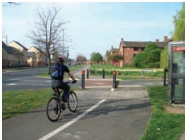
Figure 10.5 Bent-out cycle track crossing (Alex Sully)
