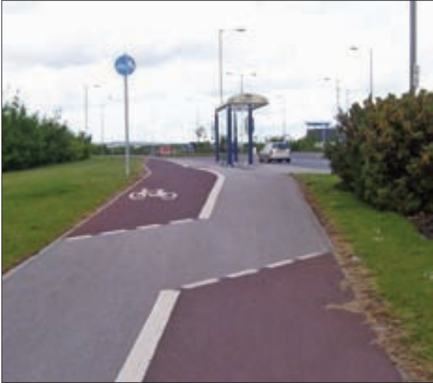
Figure 8.4 Cycle track changing sides at bus stop (Tim Pheby)
