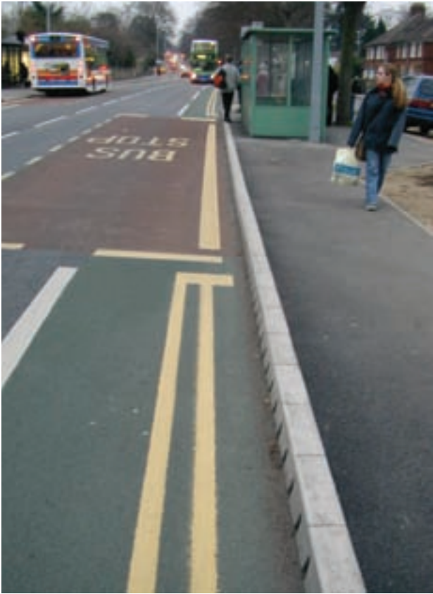
Figure 6.2 Cycle lane discontinued at bus stop (Patrick Lingwood)
