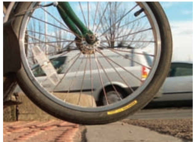
Figure 8.3 Flush surfaces at dropped kerb (Alex Sully, ERCDT)
