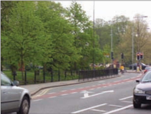
Figure 9.7 Cycle lead-in lane leading to ASL on the off-side of a filter lane (Patrick Lingwood)
