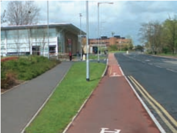
Figure 10.6 Cycle track transition to with-flow cycle lane (Patrick Lingwood)
