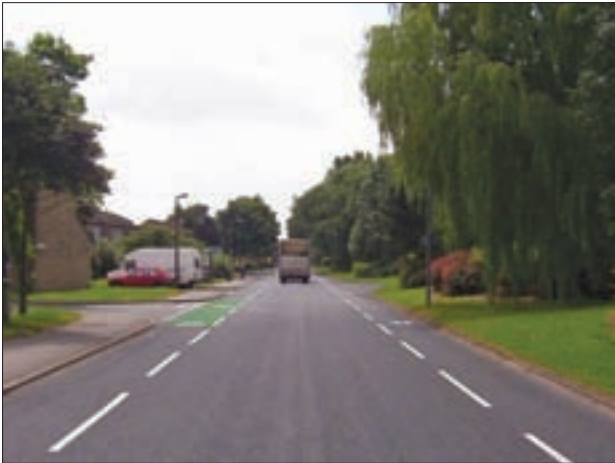
Figure 5.2 Cycle lanes on road with no centre line (Tim Pheby)
