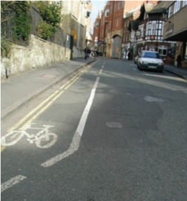
Figure 7.2 Cycle lane on uphill side of steep hill, (Patrick Lingwood)
